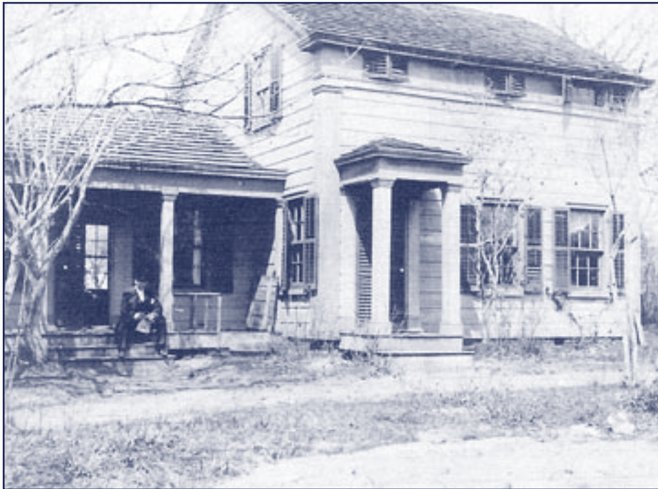
The Fraser home and studio, 249 Beaver Dam Road
