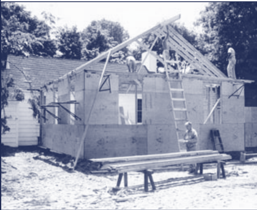
1970 addition under construction
