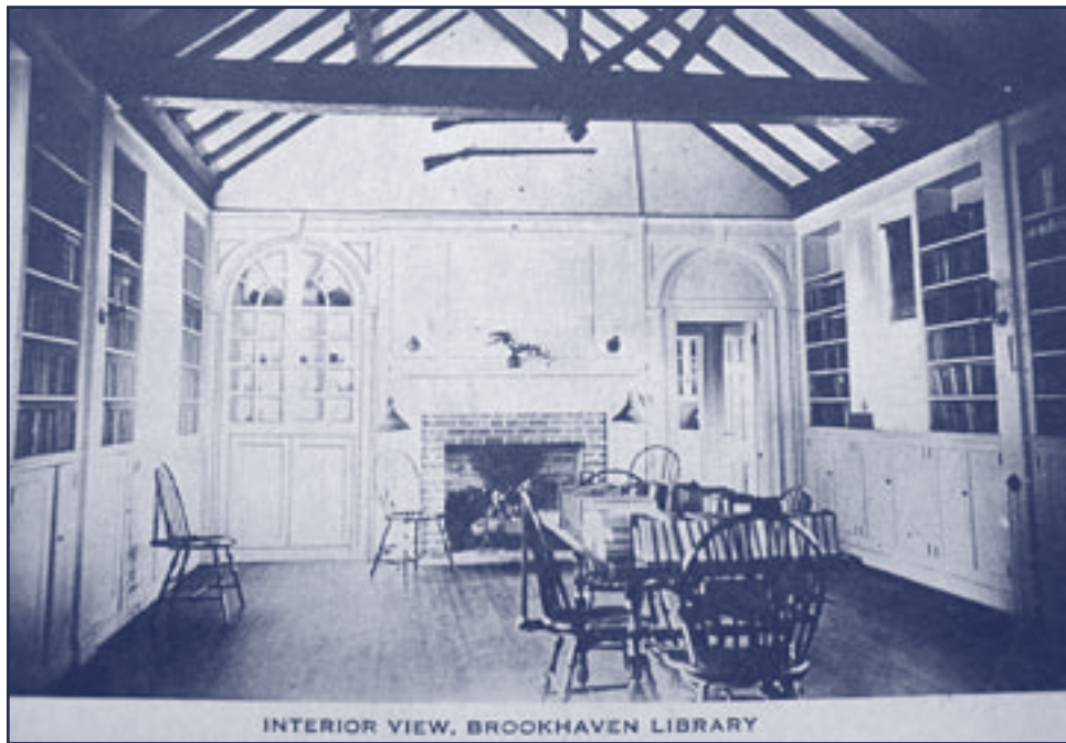
INTERIOR VIEW, BROOKHAVEN LIBRARY
